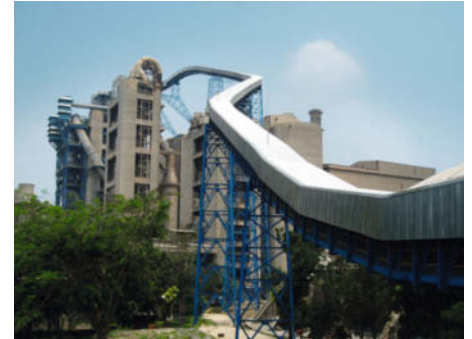
Pipe Conveyor BEUMER, Indocement, Jakarta, Indonésie
