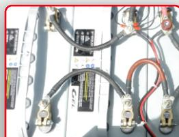
**BATTERIES : Gel 4 x 12V/76A (C5)**
