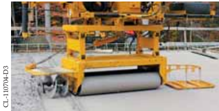
The above bridge deck is being finished on a skew using the three-point finishing system.
