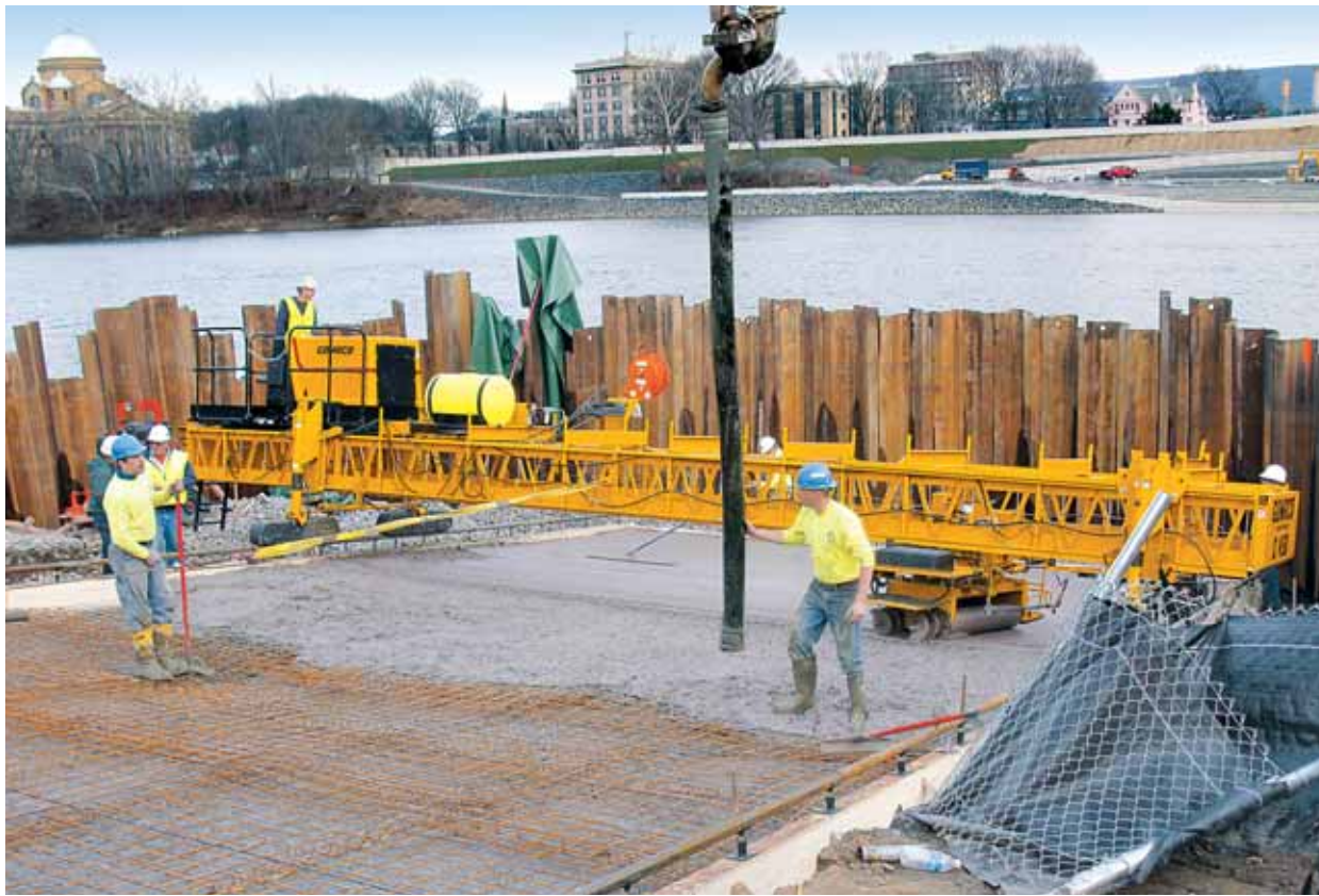
The GOMACO C-450 is finishing a unique project, a boat ramp. A coffer dam was built to keep the river back since the ramp starts at seven feet (2.13 m) below water level.
