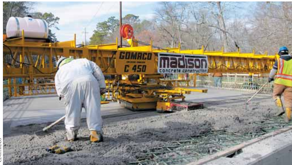
The above bridge deck is being finished on a skew using the three-point finishing system.
