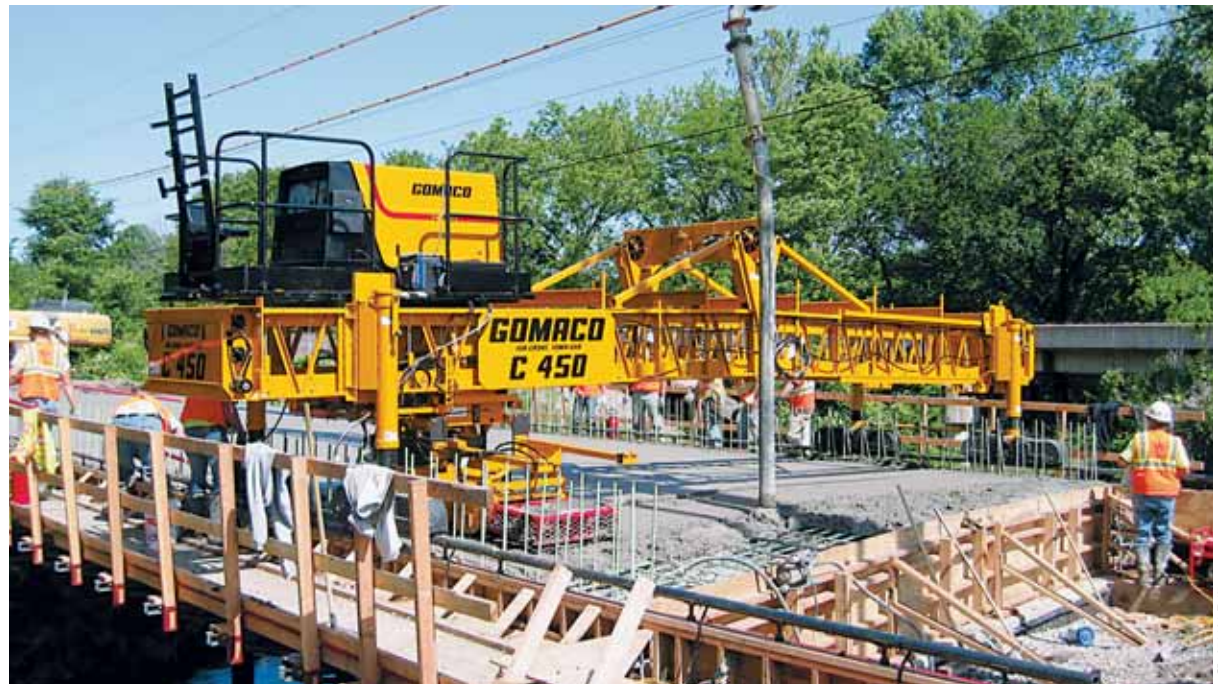
The C-450 is equipped with a power transition adjuster (PTA), allowing changes in crown elevation on-the-go, and an adjustable auger to level the concrete ahead of the finishing cylinders.
