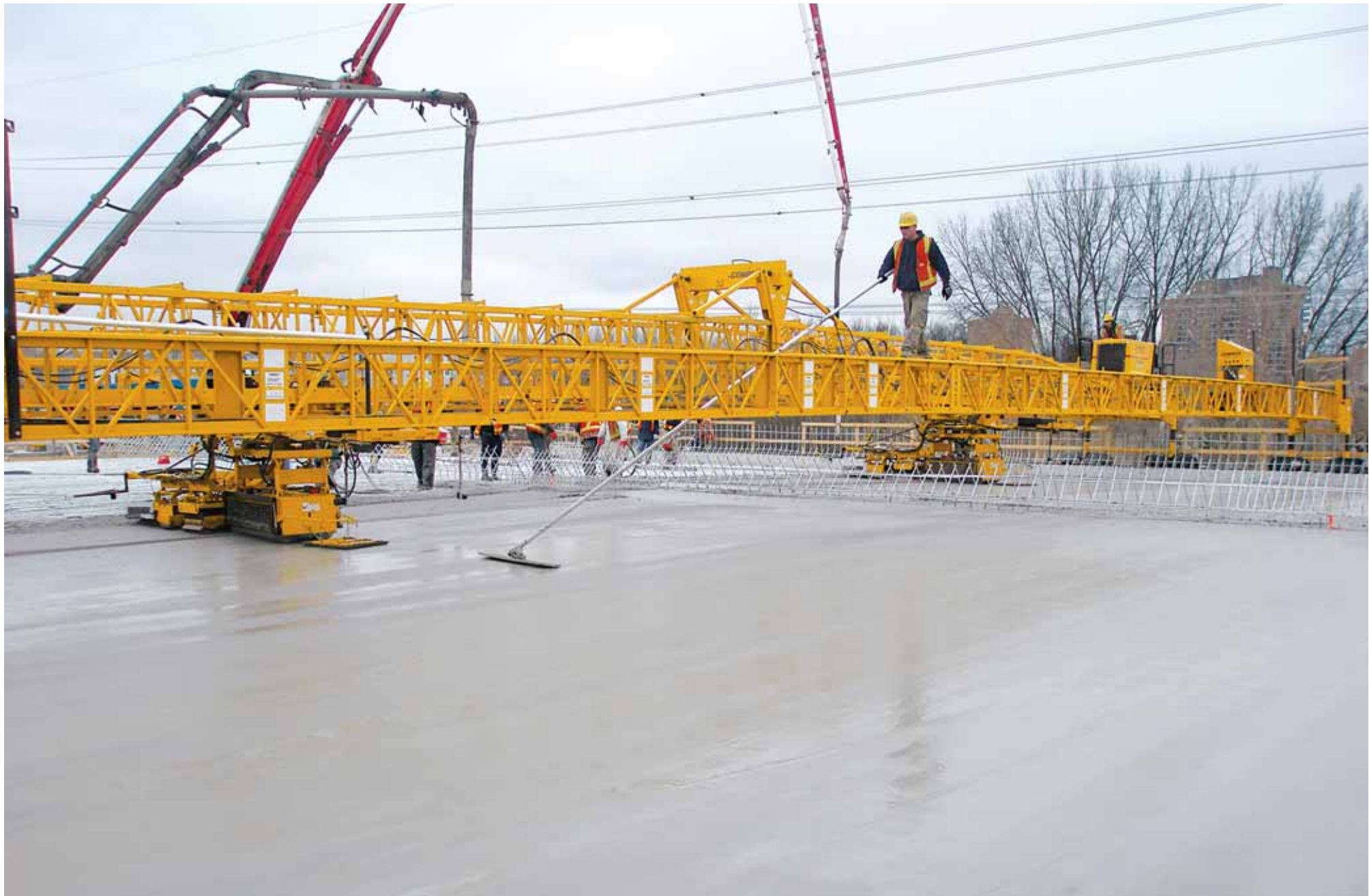
The C-450 is equipped with transitional framework and two undercarriages to finish a bridge deck. The GOMACO machine also features adjustable augers and pan-type vibrators on each undercarriage. The GOMACO cylinder finisher is followed by a powered Spanit® Work Bridge.
